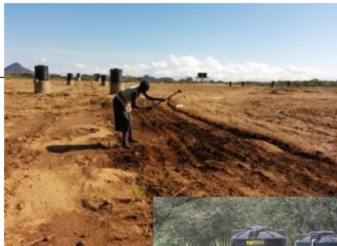
↑ A Turkana woman fills in a ditch where irrigation pipes were laid. Reservoir tanks in the background.
