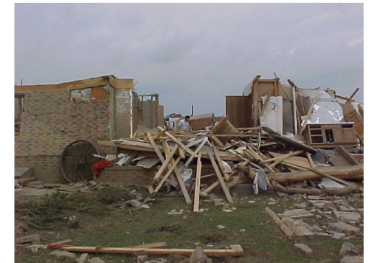
What's left of Paul and Shirley Unruh's home south of Greensburg, Kansas.
