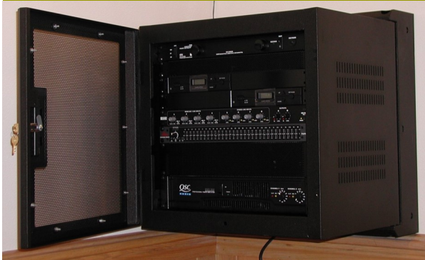
Sound system mixer and amplifier in the Little Chapel
