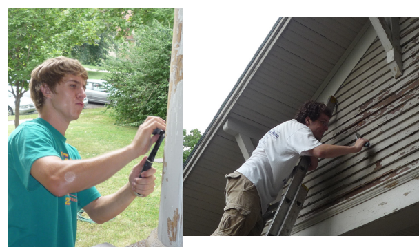
Willing volunteers helped make the Campus Ministry House possible!
