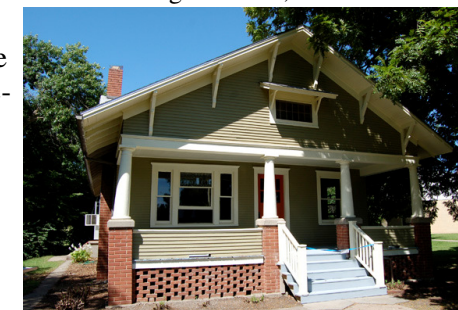
“After” picture The Campus Ministry House
