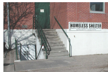
The Entrance to the Homeless Shelter, 209 E. Broadway (at the back of the building, east side)
