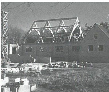
The BCMC building under construction in 1953 from the book Campus, Congregation, and Community: The Bethel College Mennonite Church 1897-1997 by Keith Sprunger
